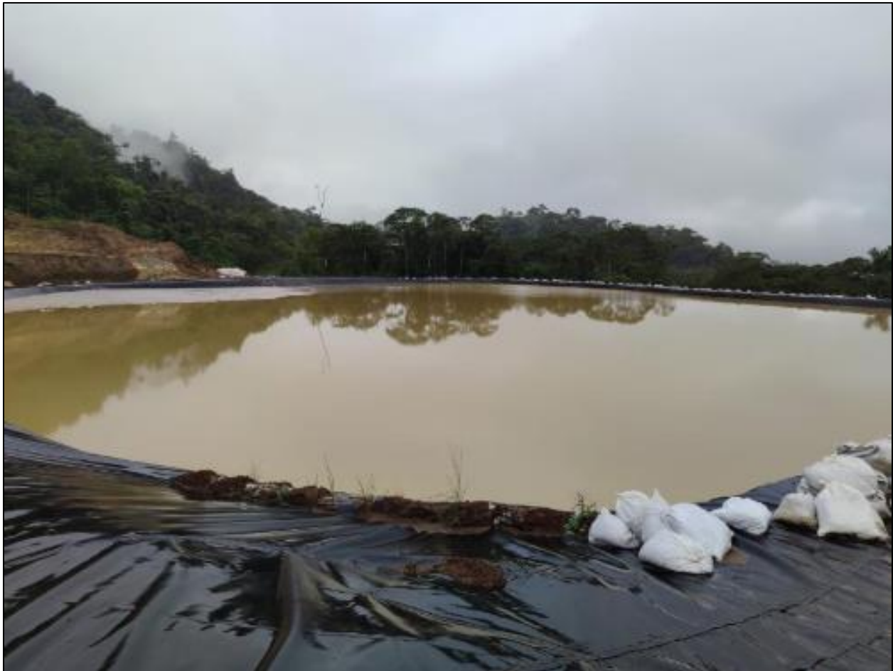
Figure 13. Pond No. 15 at the El Corazón mine contained about 50,000 cubic meters of water and tailings prior to the failure of the tailings dam on November 4, 2023. Photo from Municipio de Cotacachi (2023a).
