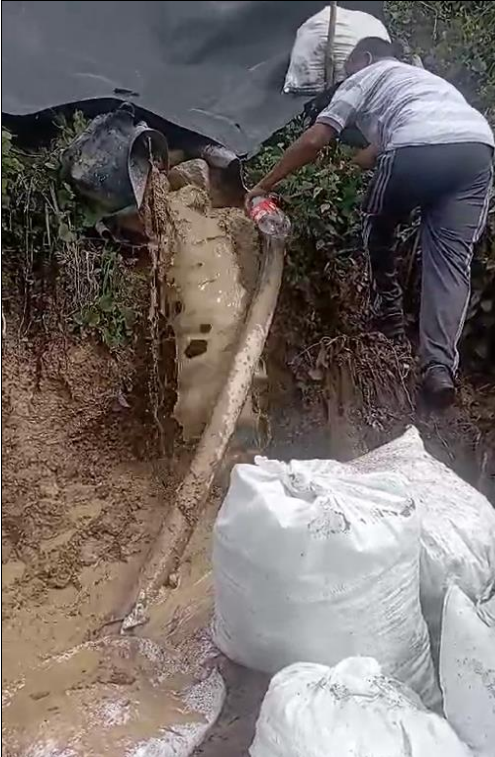
Figure 6. On the day of the tailings dam failure (November 4, 2023), a local resident struggles to gain footing on the steep embankment to collect a water sample from the leaking dam (see results of water analysis by Laboratorio Anncy (2023) in Table 1). The steepness of the embankment is further indicated by the steepness of the pipe, the exposed plant roots, and the near vertical fall of contaminated water from the tailings pond. Still photo at 0:04 of video provided by Asociación de Propietarios de Tierras Rurales del Norte and Frente Antiminero (labeled Video 1 by author). Another still photo from the same video is available in Municipio de Cotacachi (2023a).
