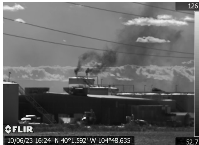
Uncontrolled release of hydrocarbons from a storage tank at an oil and gas facility in Brighton, CO
