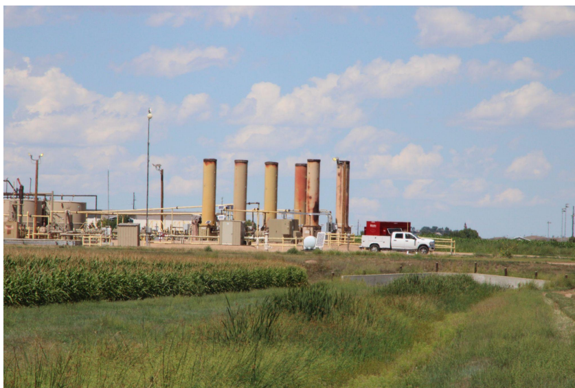
Photo of row of ECDs on Extraction Kodak well pad in Windsor, CO
