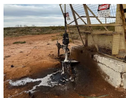
A leaking abandoned well in New Mexico.
