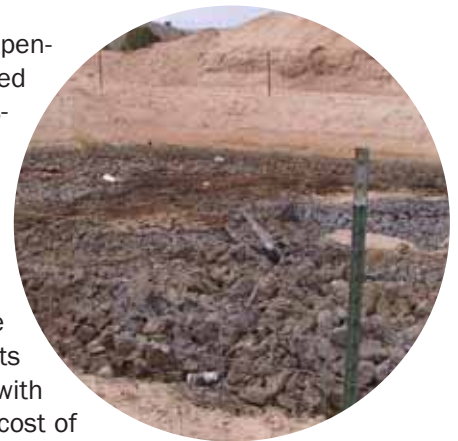
FIGURE I-6. DEWATERED DRILLING MUD Is often buried on-site.
