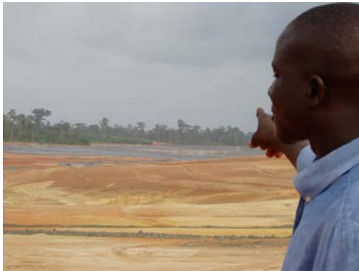
Photo 6: Independent experts have questioned why Newmont did not fully line the Ahafo mine's tailings dam, where waste will be stored, to reduce the risk of contamination.
