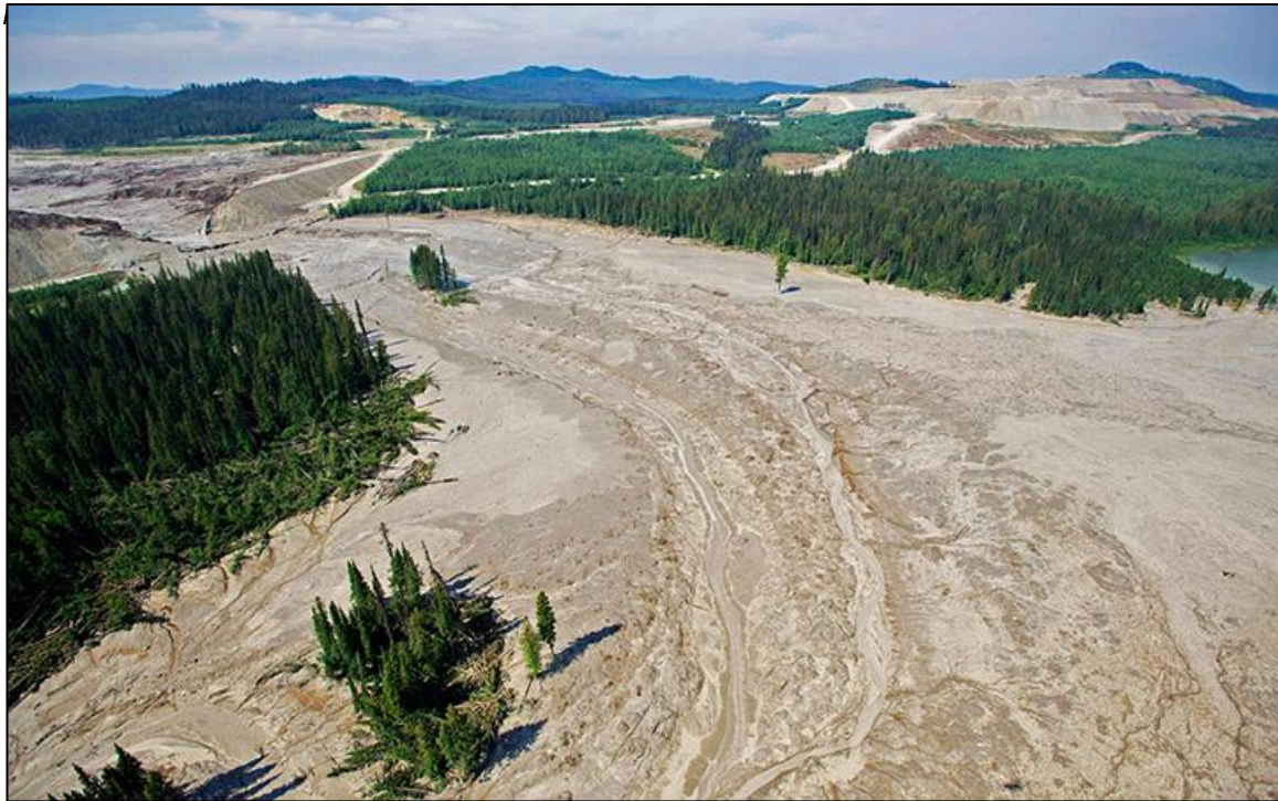
Mine tailings flow from tailings dam failure at Mount Polley Mine.
