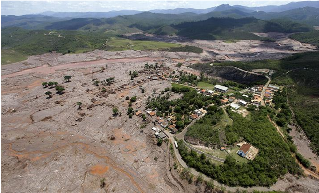
Samarco tailings dam failure, Brazil, 2015
