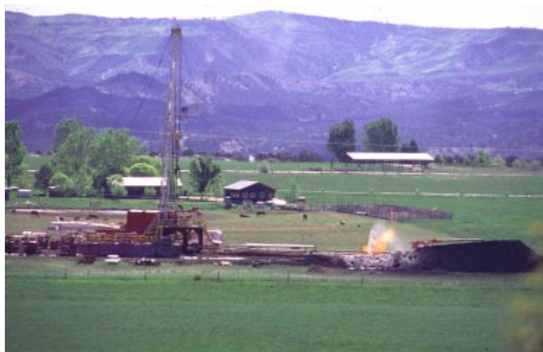
Oil and gas wells and their impacts on rural communities in the West. Depicted here, the stimulation of a newly drilled well by cavitating and flaring tons of coal and drilling wastes. Taken near Durango, Colorado, May 2001.
