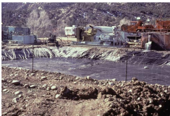
This reserve pit is designed to hold wastes while work is being done on the well. The plastic used to line the pit is often torn, allowing contaminants to seep into soils and groundwater.
