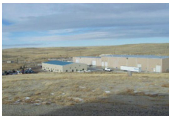
Smith Ranch-Highland facility. Photo source: NRC
