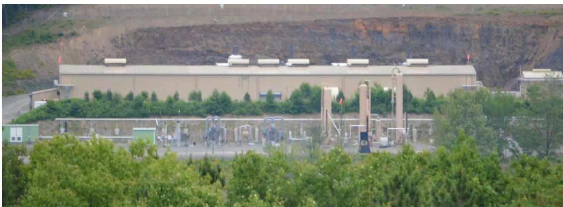
Dunbar Compressor Station, Broome County, New York. Photo by Earthworks.
