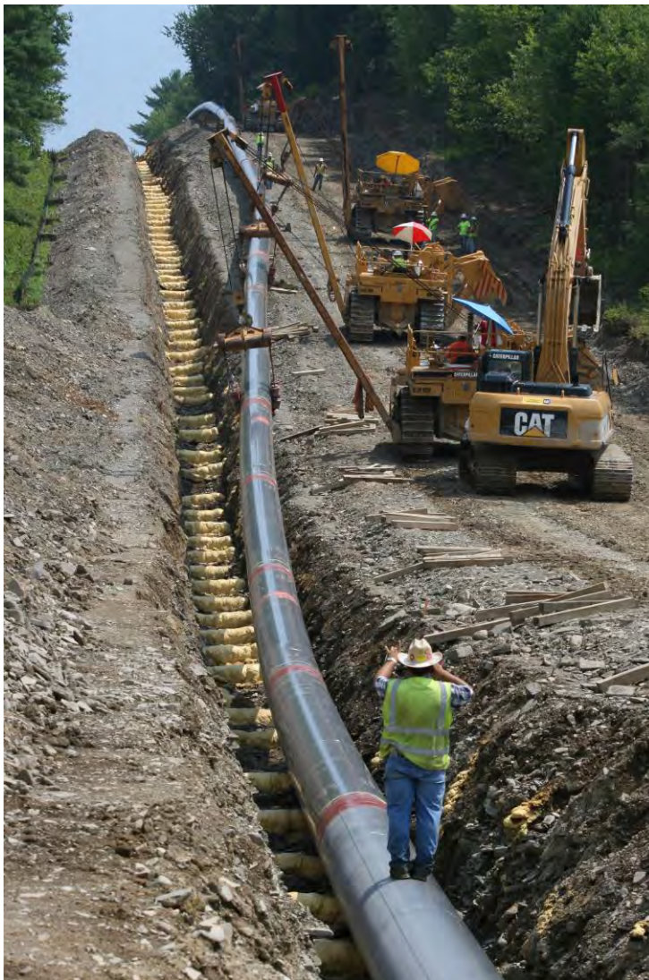
Forest cut for construction of the Millennium Pipeline, Broome County, New York. Photo by Roger Luther, nyslandmarks.com.
