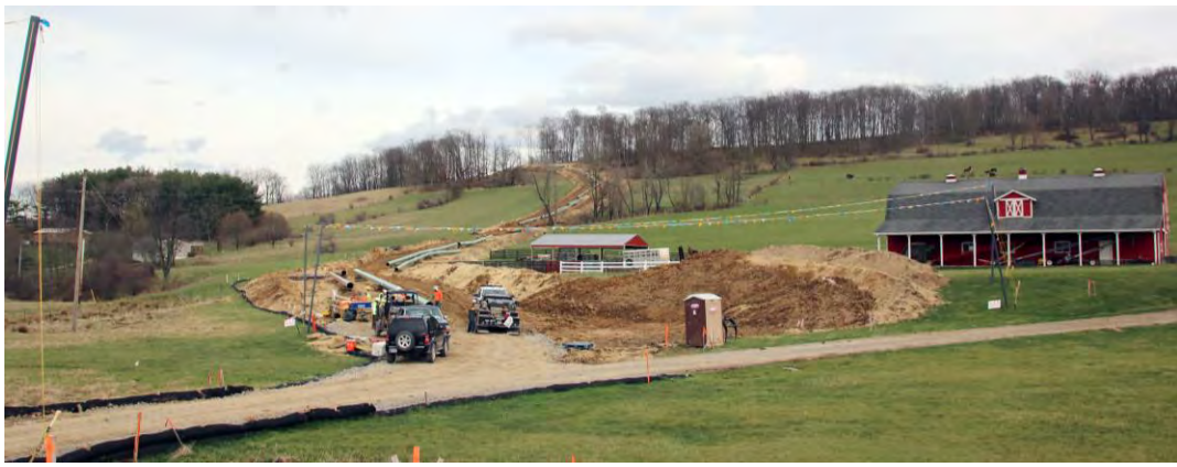
Pipeline construction, Washington County, Pennsylvania. Photo by Earthworks.
