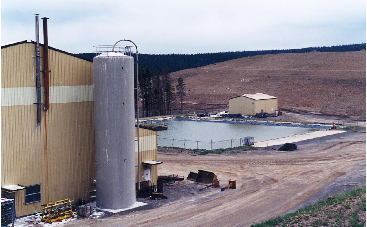
Water pollution from the Beal Mountain Mine near Anaconda requires costly treatment.
