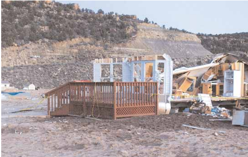
FIGURE II-8. REMAINS OF A TRAILER IN LA PLATA COUNTY, CO. The trailer exploded due to methane that most likely came from an inadequately plugged orphan well. Photo Credit: Yodit Gidey, Durango Herald.
