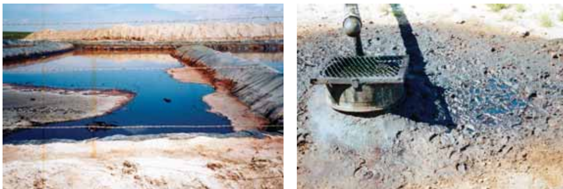
FIGURE I-32. SOUTHEAST NEW MEXICO: Left: produced water pit with layer of oil on top. Right: Leaking waste-oil tank. No netting and inadequate fencing allows access to these toxic hydrocarbon wastes. Photo by C. Johnson.
