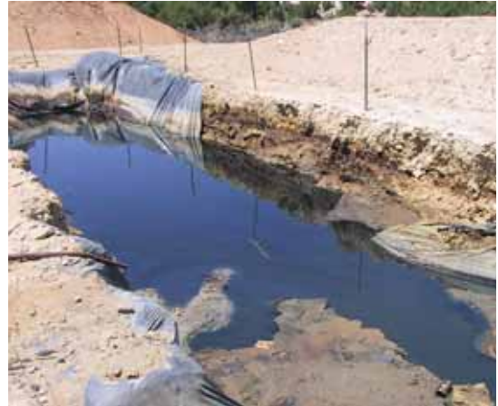
FIGURE I-21. TORN LINER ON AN OPEN PIT.
