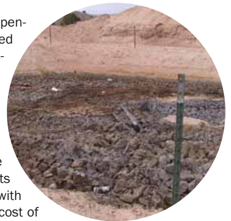
FIGURE I-6. DEWATERED DRILLING MUD Is often buried on-site.
