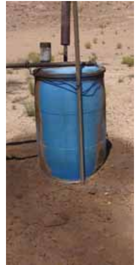
FIGURE I-33. LEAKING TANKS CAN THREATEN GROUNDWATER. Note the hydrocarbon stains on the soil.
