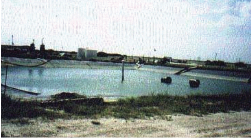
ISL Evaporation Pond
