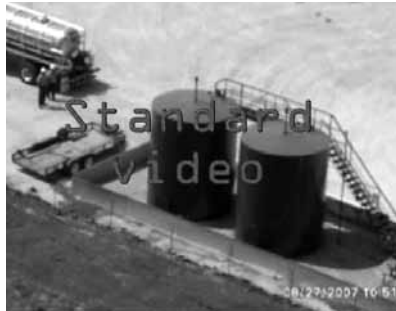
Before: Well without the benefit of infrared to capture fugitive emissions.
