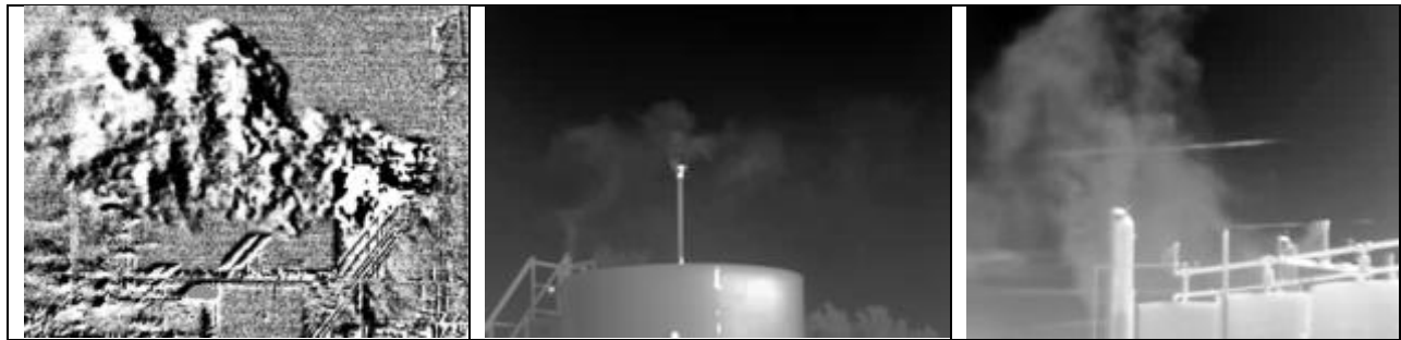
Above: significant tank vapor emissions within the RMP-A planning area.
