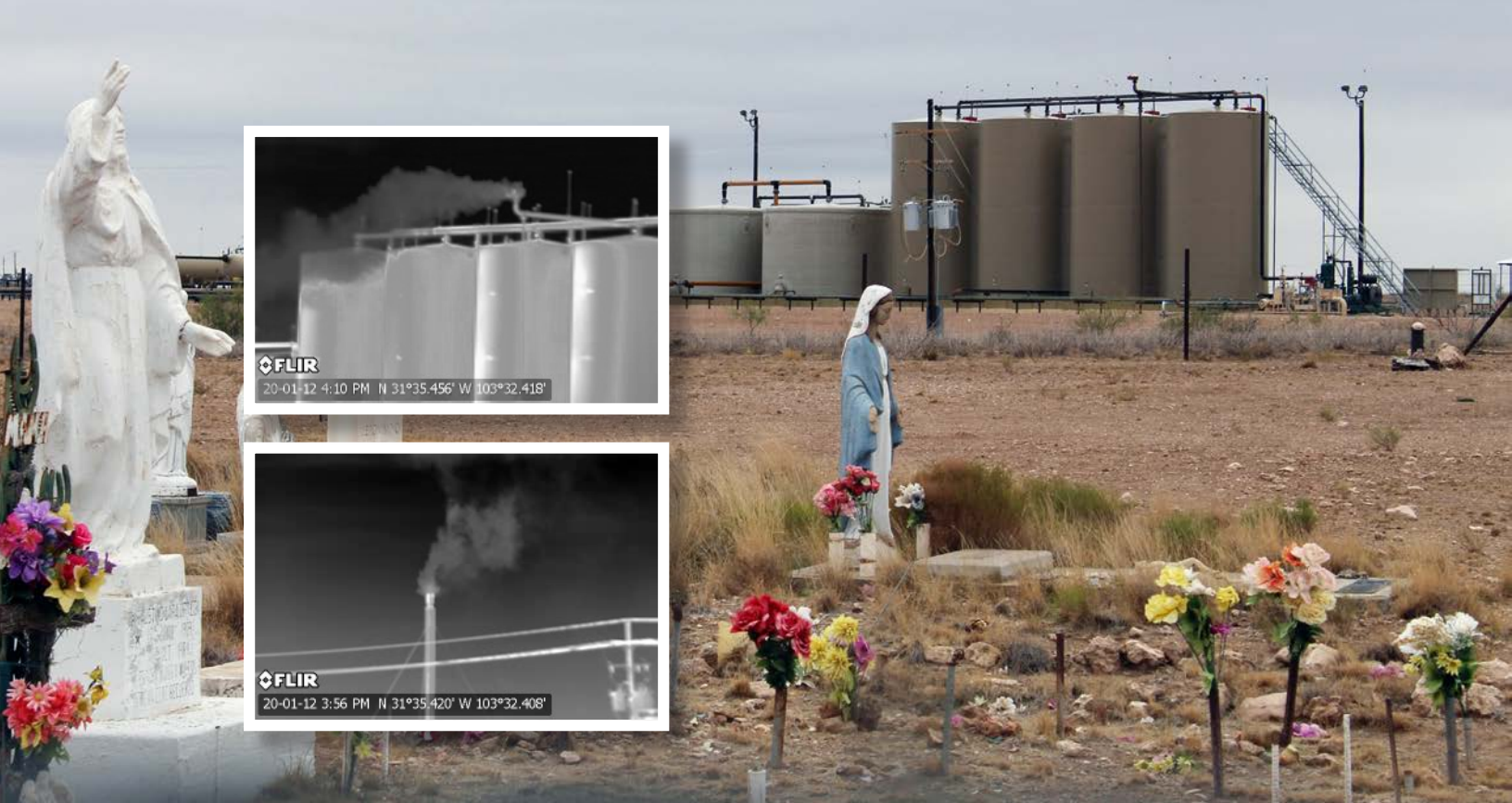
Below, the Diamondback Misbehaving well is on General Land Office land and within sight of a cemetery. Inset Optical Gas Images from on site: Upper shows a tank venting significant hydrocarbon emissions. Lower shows hydrocarbons released by an unlit flare.
