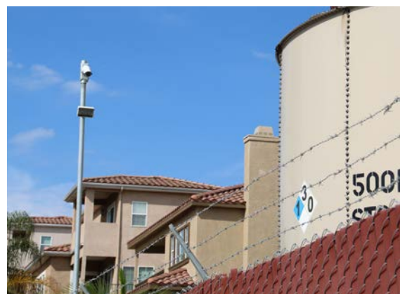
Oil tanks close to homes in Los Angeles County.
