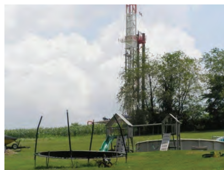
Drilling directly behind the play yard.
