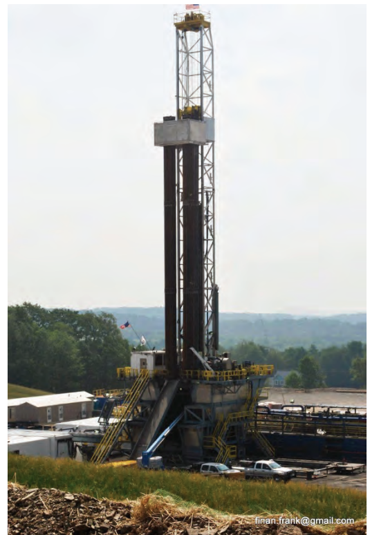
Drilling rig onsite.
