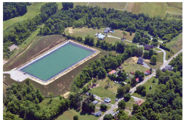
Impoundment pits, which often contain contaminated waste, can leak and give off emissions.
