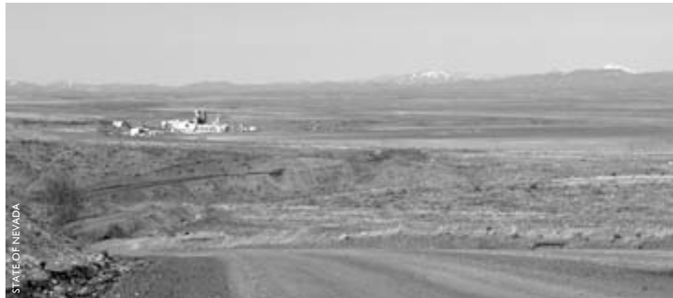
In 2004, Nevada's Jerritt Canyon Mine was the single largest emitter of airborne mercury in the US.
